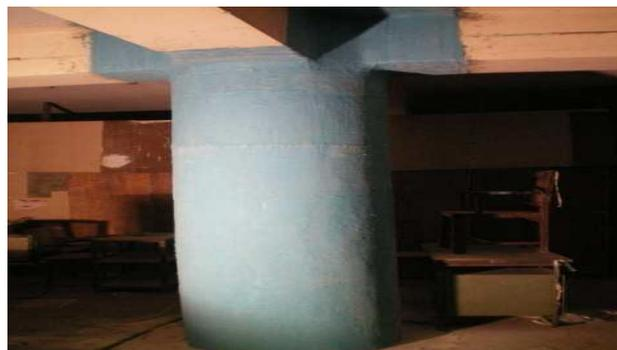
**Figure 3: Final look of column after plastering**
