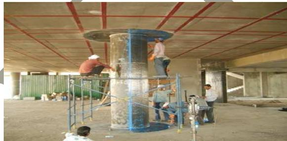
**Figure 2: Cutting and applying of fiber sheet on the column**
