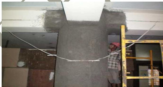
**Figure1: Surface grinded and prepared for fiber wrapping**
