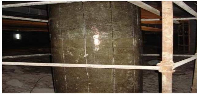
**Figure 1: Surface Primer applied on the column**
