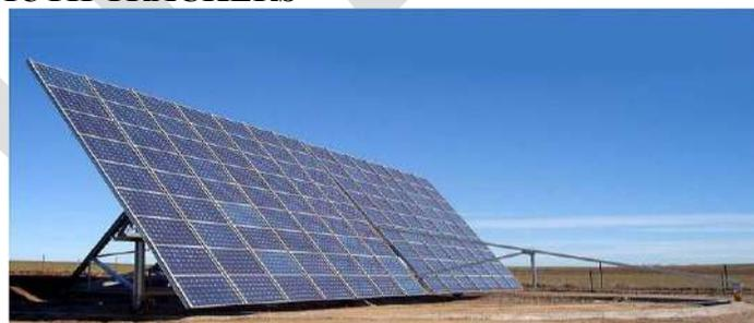
**Fig: 1.5.2.d) Altitude- Azimuth Type Tracker**
