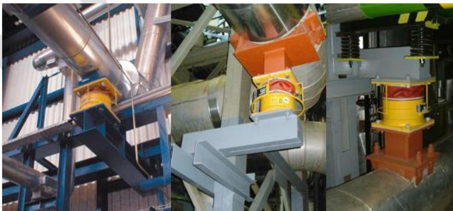
**Fig 8 Viscoelastic Damper**
