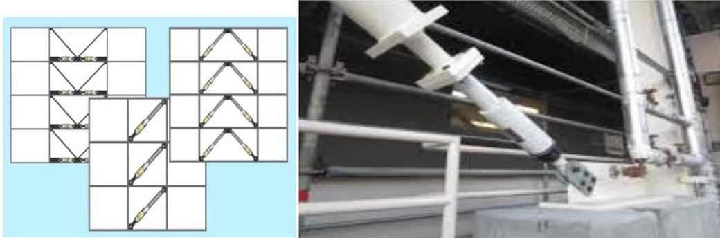
**Fig 6 Friction Damper**
