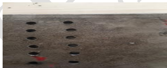
Holes drilled under HPCJ Condition
