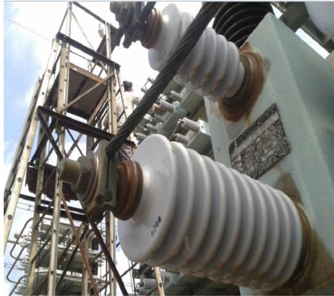
**Fig 1.2 Filter capacitor bank without Lug**
