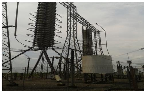
**Fig. 1.4 Bird fault frequently occurs on this filter banks**
