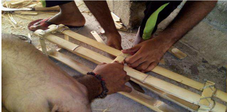
Fig 2.1 Preparation of bamboo reinforcement cage
