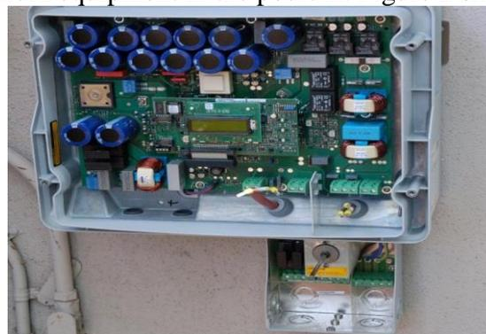
**Figure 2: Solar Inverter**
