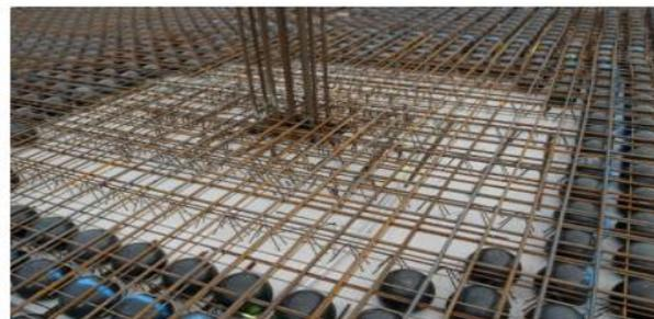
Fig-3 Placing of Bubble<sup>[4]</sup>
