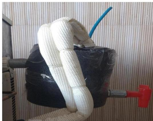
Photograph 3 Cold water storage tank
